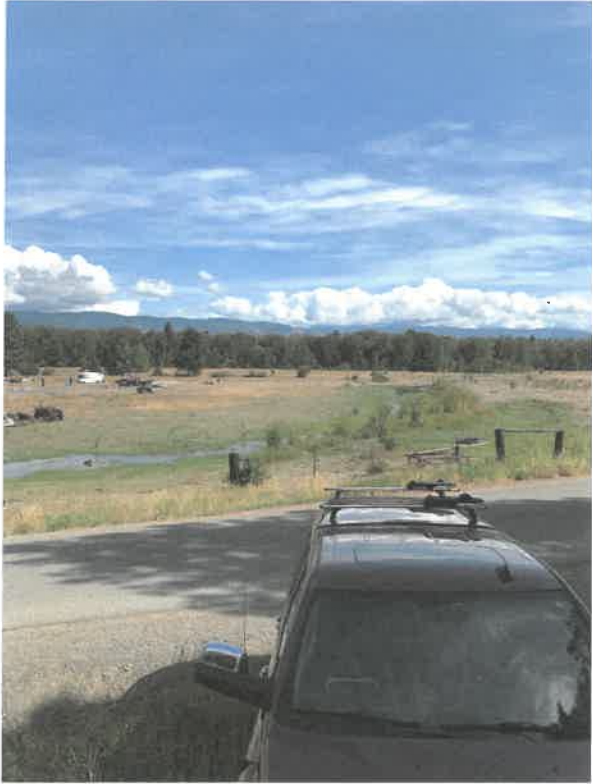
Existing Infrastructure – Parcel 20474
